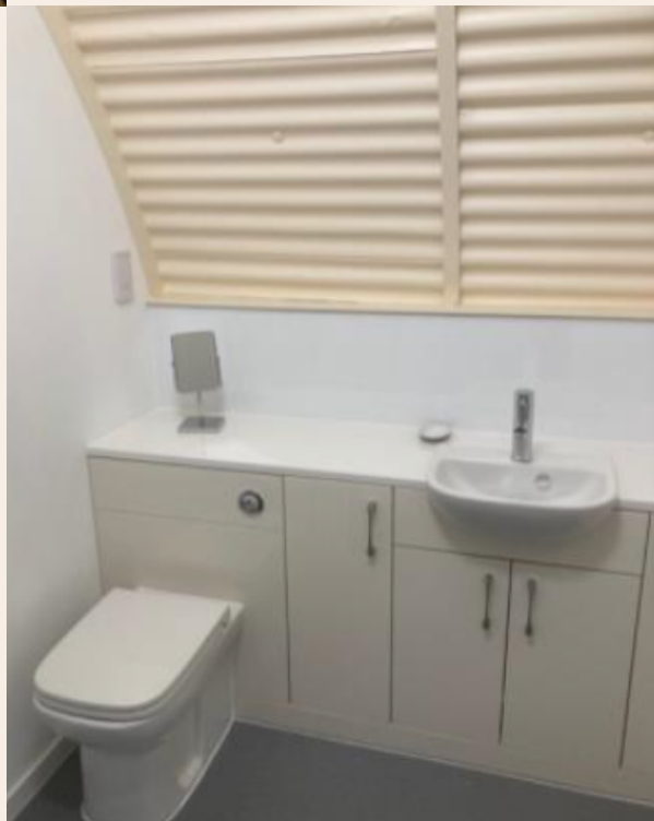
Example of bathroom installation in recently refurbished Grade B self-catering hut
